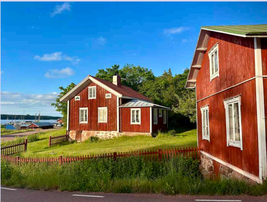
Photo: Nordic Sustainable Construction, picture from Åland
