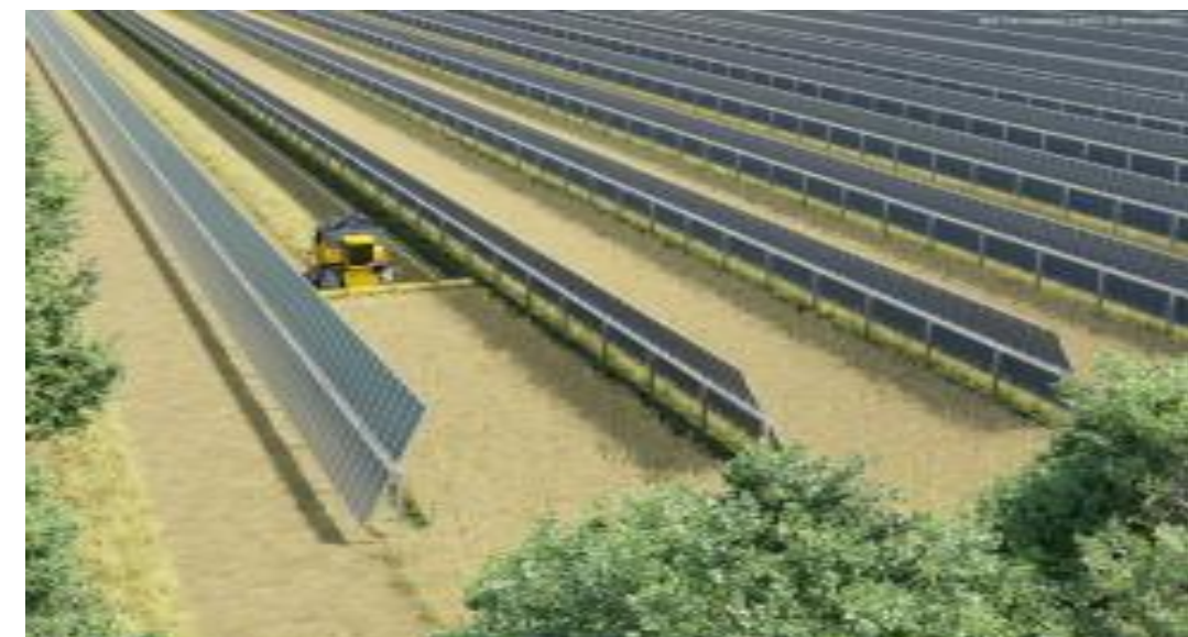
Fig 1: Agri-PV system with wide row spacing, allowing sunlight to reach crops and enabling easy access for agricultural machinery between solar panel rows—illustrating effective dual land use for farming and clean energy production.
