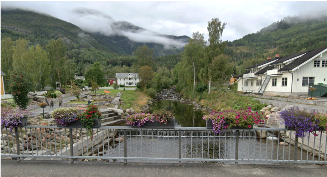
Figure 4 Retention basin, Nesbyen Norway
