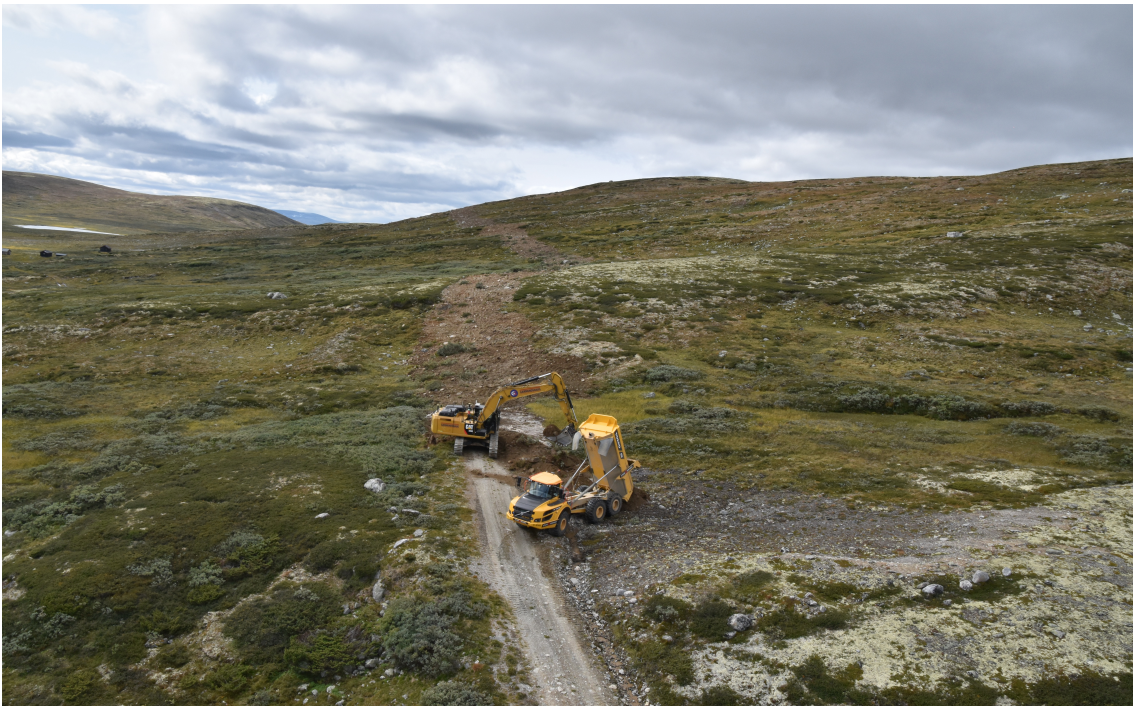
Figure 16. Road removal and restoration of a shooting range at Hjerkin, Dovrefjell in Norway. Photo: Dagmar Hagen.
