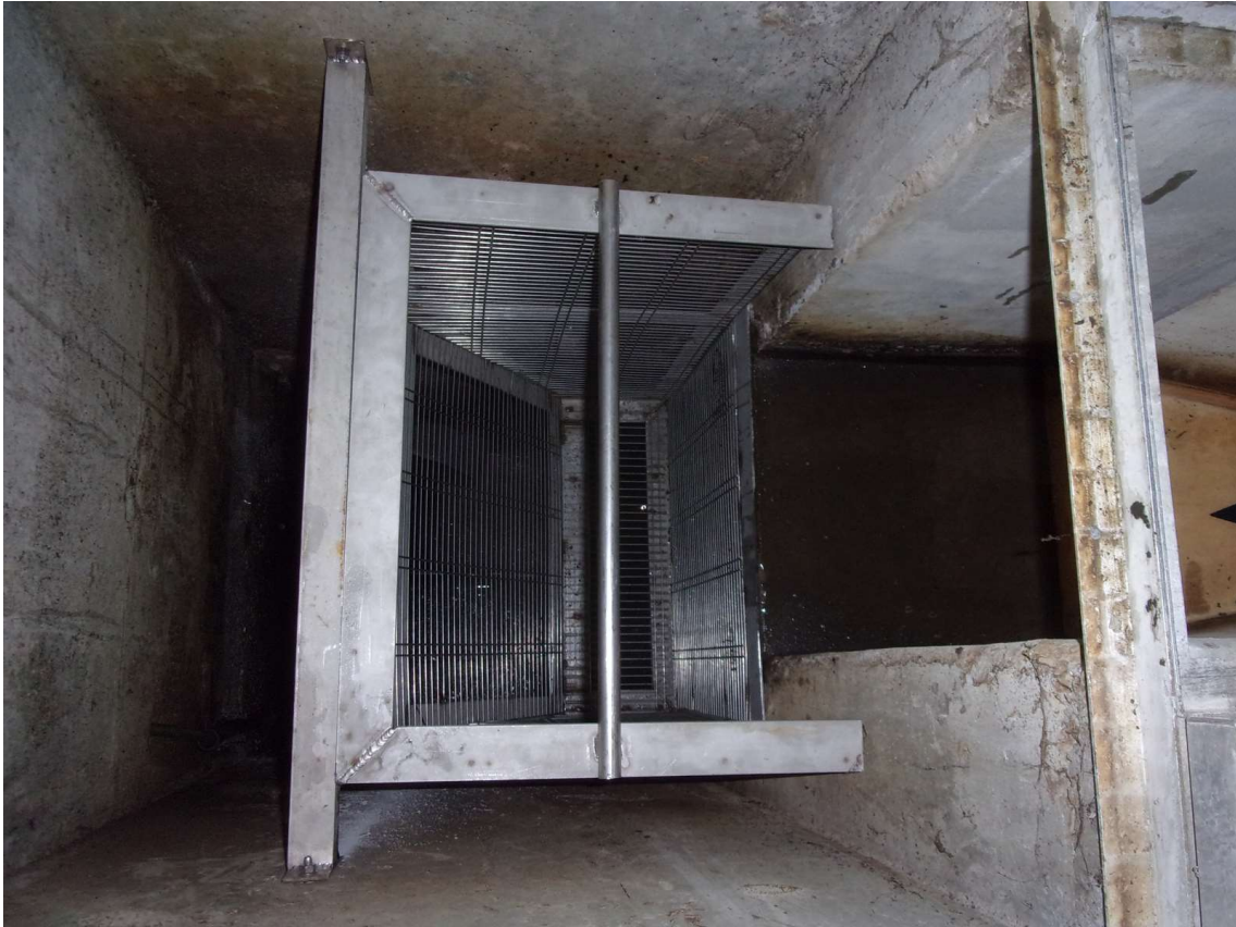
Figure 6 Installation of grids at an overflow© AcquaPublica
