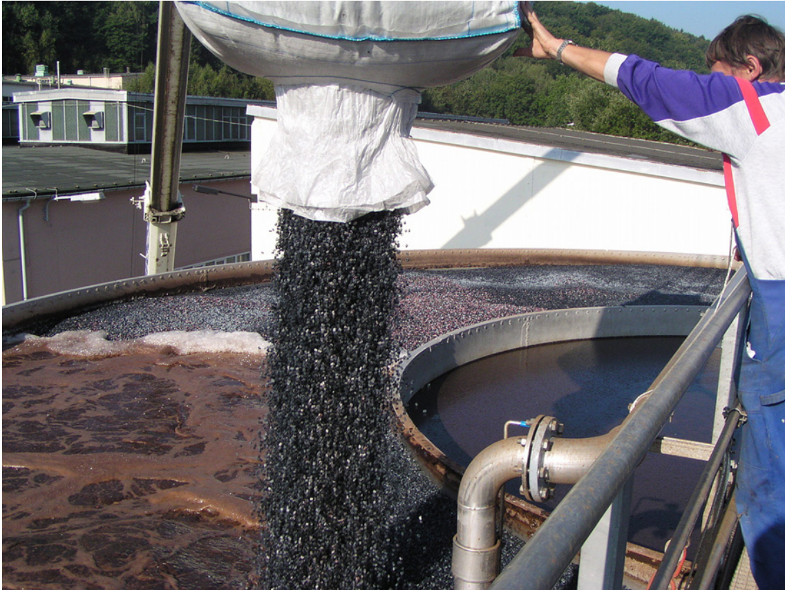
Figure 8 Safe pouring of biocarriers into an open tank ©Mutag
