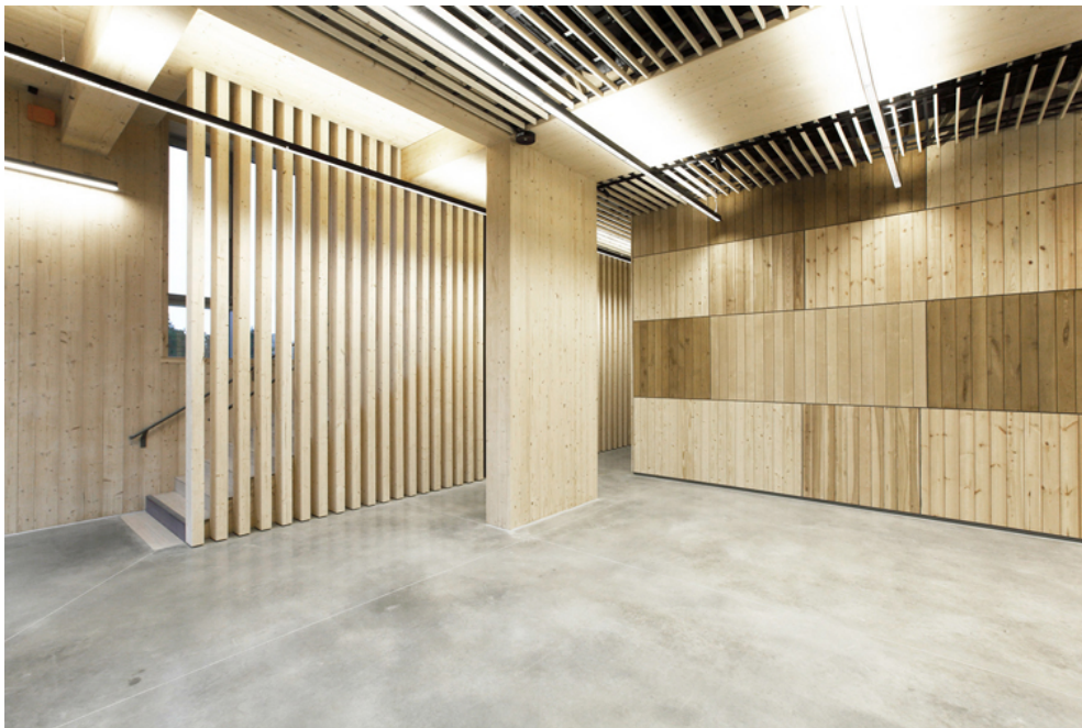
Figure 30. New extension has a load-bearing timber frame that is partly exposed to the interior. Photo: Tõnu Laigu
