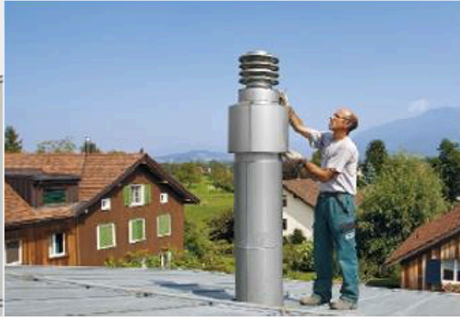
Figure 7a: ESP fitted at the mouth of the chimney
