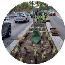
Nacka: Transforming a large road to meet a new urbanisation context
